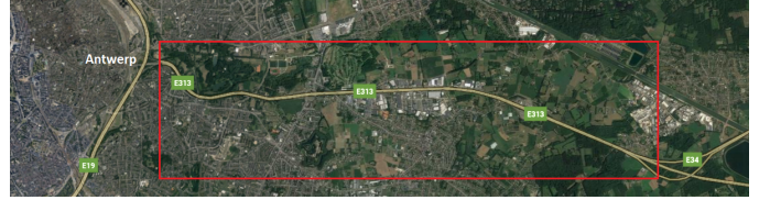
Fig. 7: The segment of the two way E313 highway in Antwerp, Belgium. © 2020 Google.
